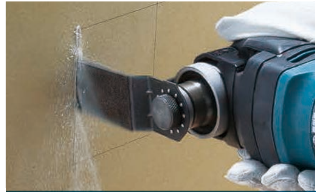
Cutting plasterboards
