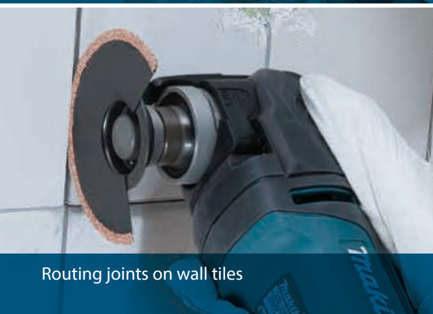
Removing mortar, tile adhesive
